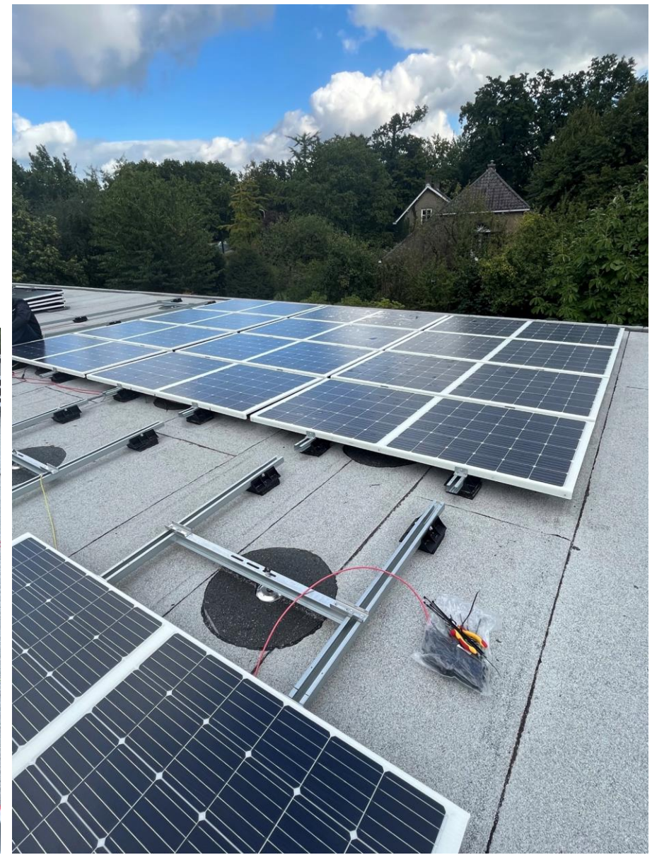
Roof parallel mounting on flat roof with roofing anchors
