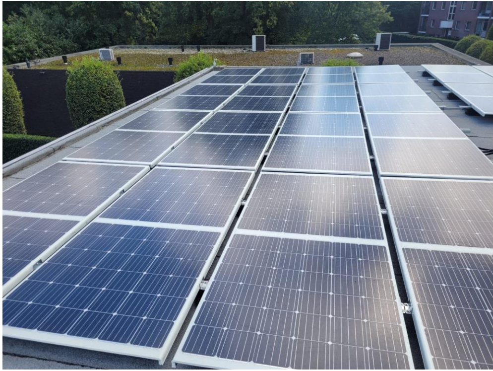
Roof parallel mounting on flat roof with roofing anchors
