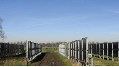
Culemborg Fixed, vertical interspace agrivoltaic system with pasture
