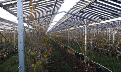
Wadenoijen Fixed, overhead agrivoltaic system with berry cultivation
