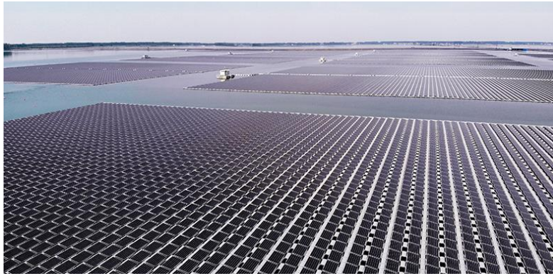
150 MW Guqiao - China
