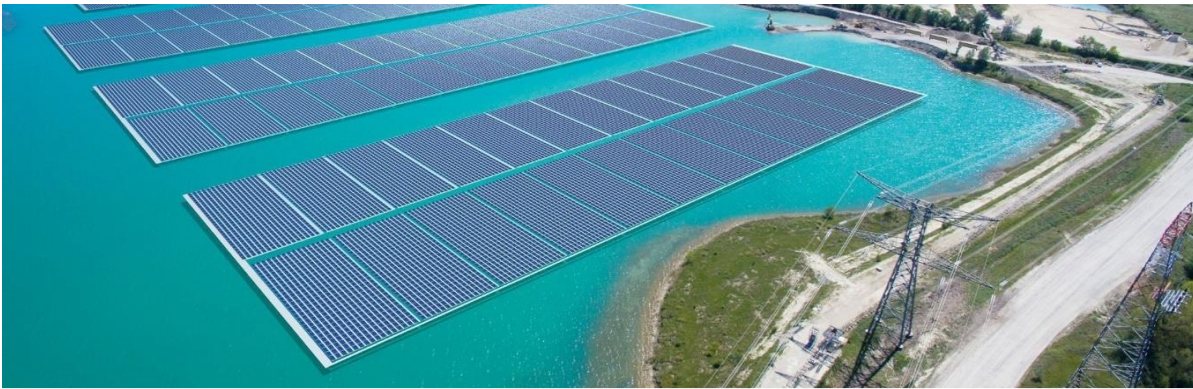
17 MW Piolenc - FR (under construction)
