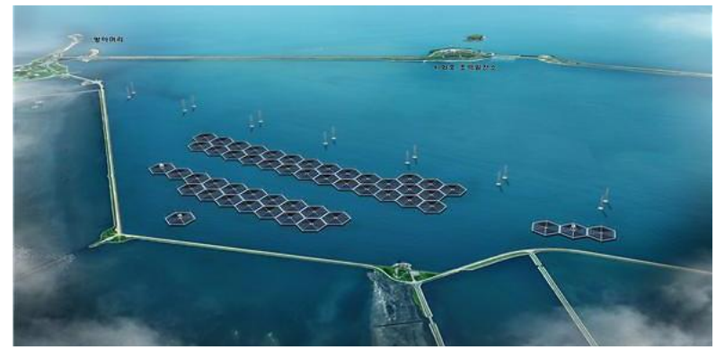
103 MW Shihwa Lake - South Korea
