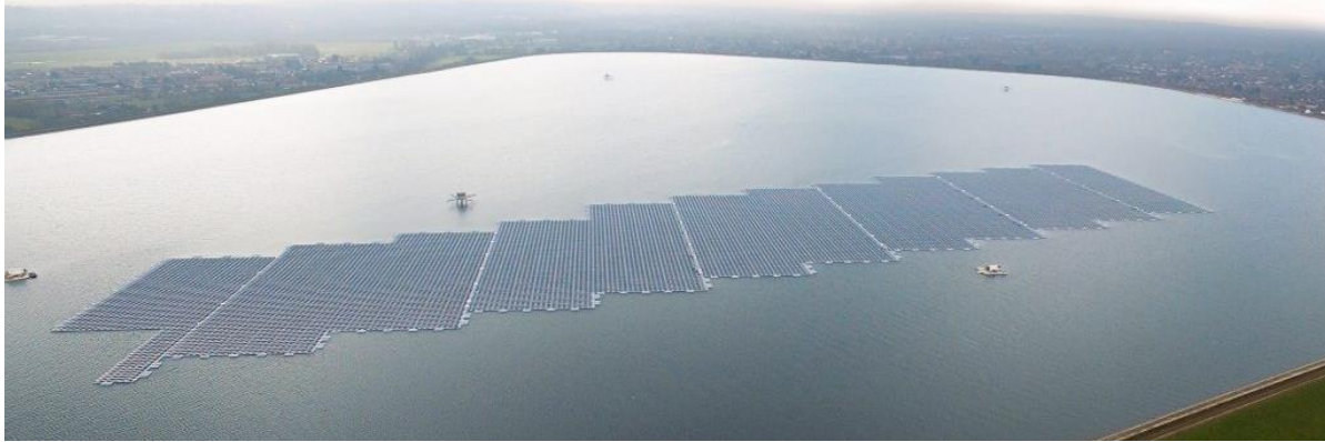
6.4 MW Queen Elizabeth II - UK (completed March 2016)
